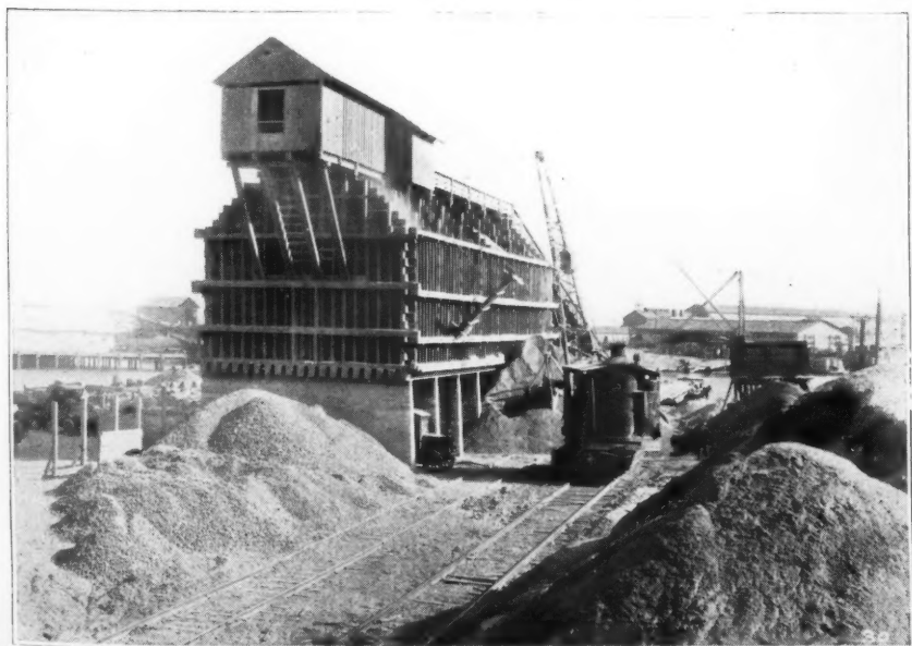
The Storage Bins and Yard Storage at Long Beach
